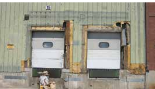
Loading dock bay door frame repair and replacement
