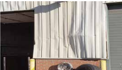
Damage restoration of panel and roll up door frame
